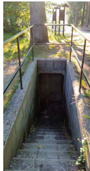
Photo: The Belveder Route – the entrance into the bunker/pillbox
